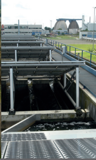
Mannheim wastewater treatment plant, filter with GAC
