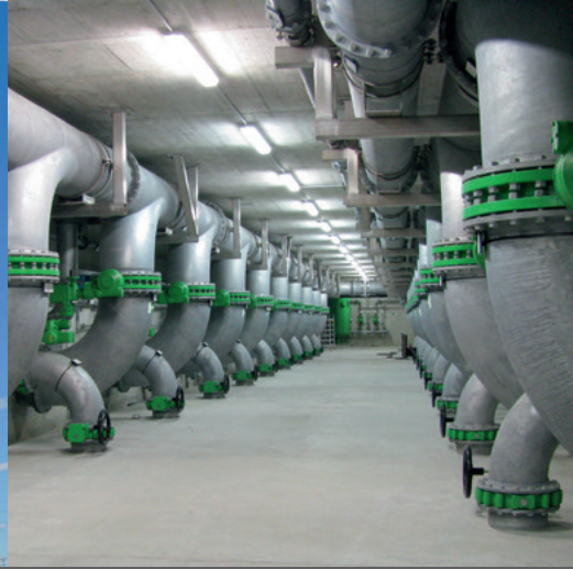
Breisgauer Bucht wastewater treatment plant Pipe system of the sand filtration stage
