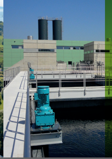
Steinhäule wastewater treatment plant, Neu-Ulm
