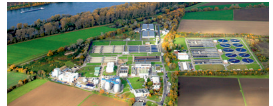
Wastewater treatment plant at Mannheim am Rhein
