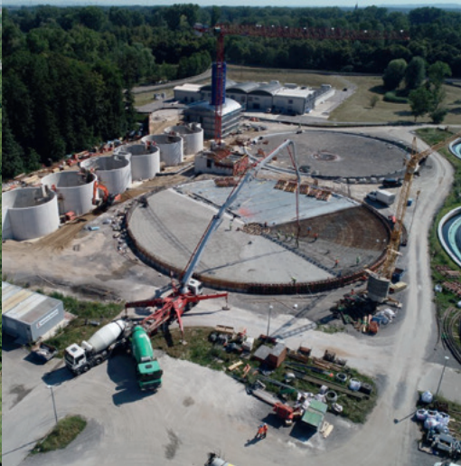
Karlsruhe wastewater treatment plant, advanced treatment stage under construction
