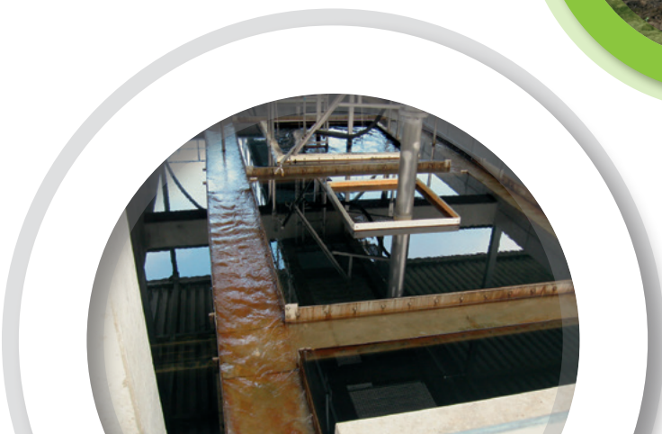
Sedimentation at the Stockacher Aach wastewater treatment plant
