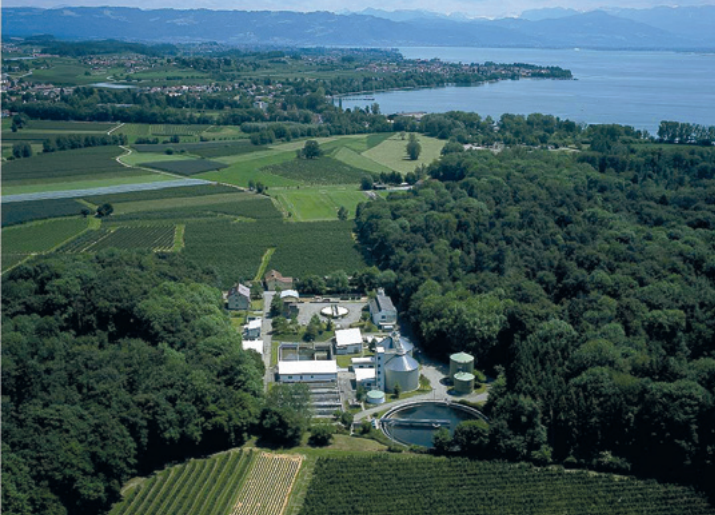
Kressbronn wastewater treatment plant located at Lake Constance and equipped with a treatment stage for targeted micropollutant removal
