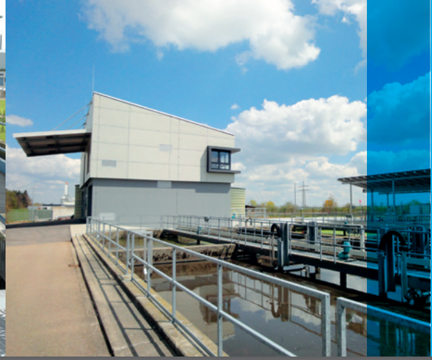
Laichingen wastewater treatment plant with activated carbon and downstream cloth filter
