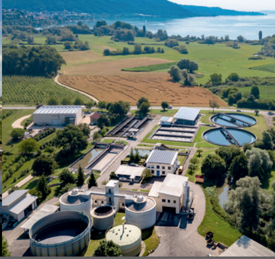
Stockacher Aach wastewater treatment plant at Lake Constance
