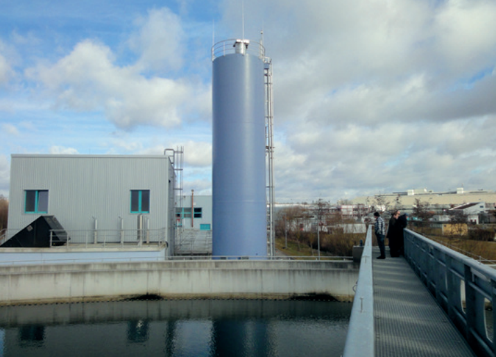
Böblingen-Sindelfingen wastewater treatment plant Adsorption stage using PAC
