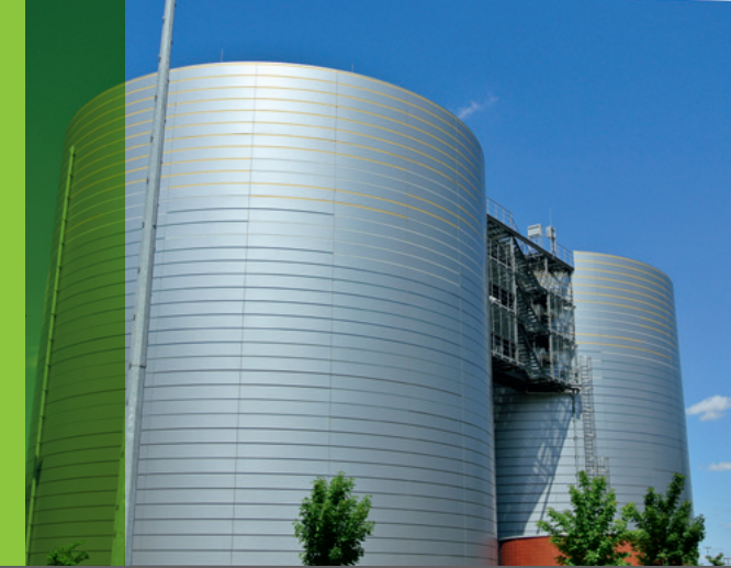
Stuttgart-Mühlhausen wastewater treatment plant
