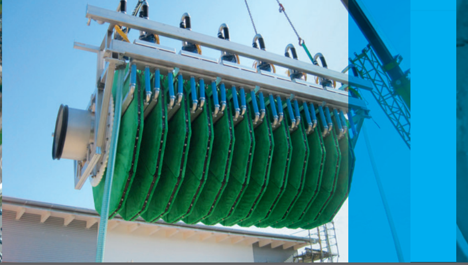
Lahr wastewater treatment plant, installation of a new pile cloth filter
