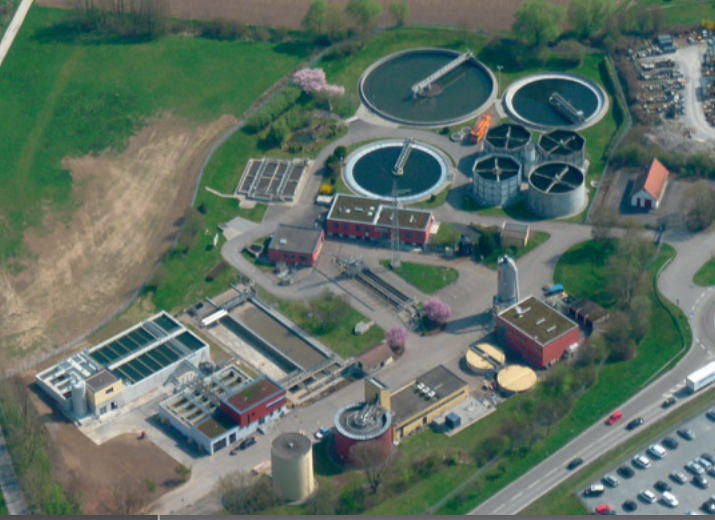
Öhringen wastewater treatment plant, using powdered activated carbon
