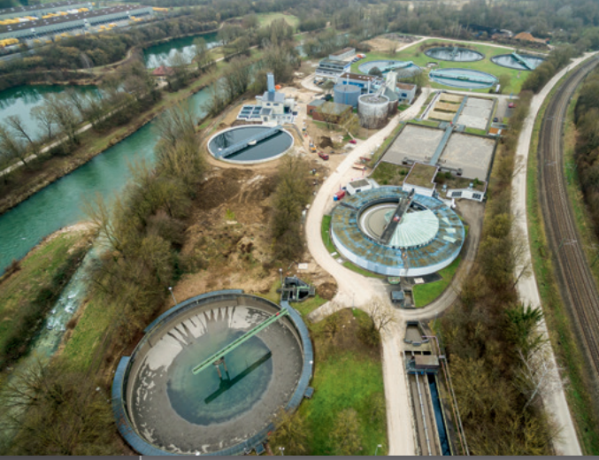
Wastewater treatment plant in Wendlingen am Neckar after completion of the powdered activated carbon-based treatment stage
