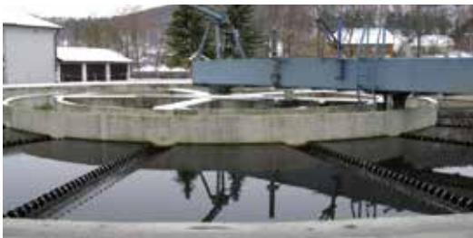
Figure 2: Sedimentation tank (former cyclator)
